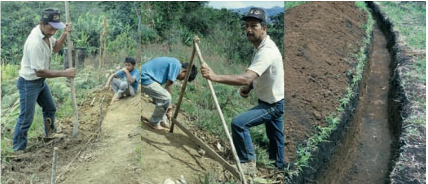
A local promoter, a land user who was trained by the Research Centre CISEC to extend the agroforestry system within the approach area, demonstrates different steps of technology implementation: demarcation of the contour lines using A-frame, pegs and rope, and digging of an infiltration ditch. His son, who is assisting, will soon learn about, and practice, sustainable land management practices at the rural college, which was established and is managed through the programme. (Mats Gurtner)
